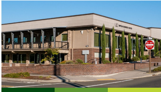
Umpqua Business Center, 522 SE Washington Ave., Roseburg
