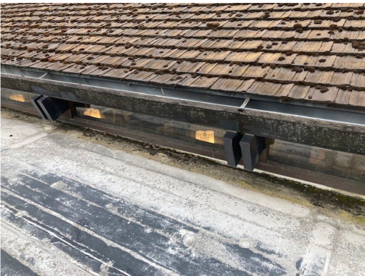
8. North Side (over bathrooms) window to remove
