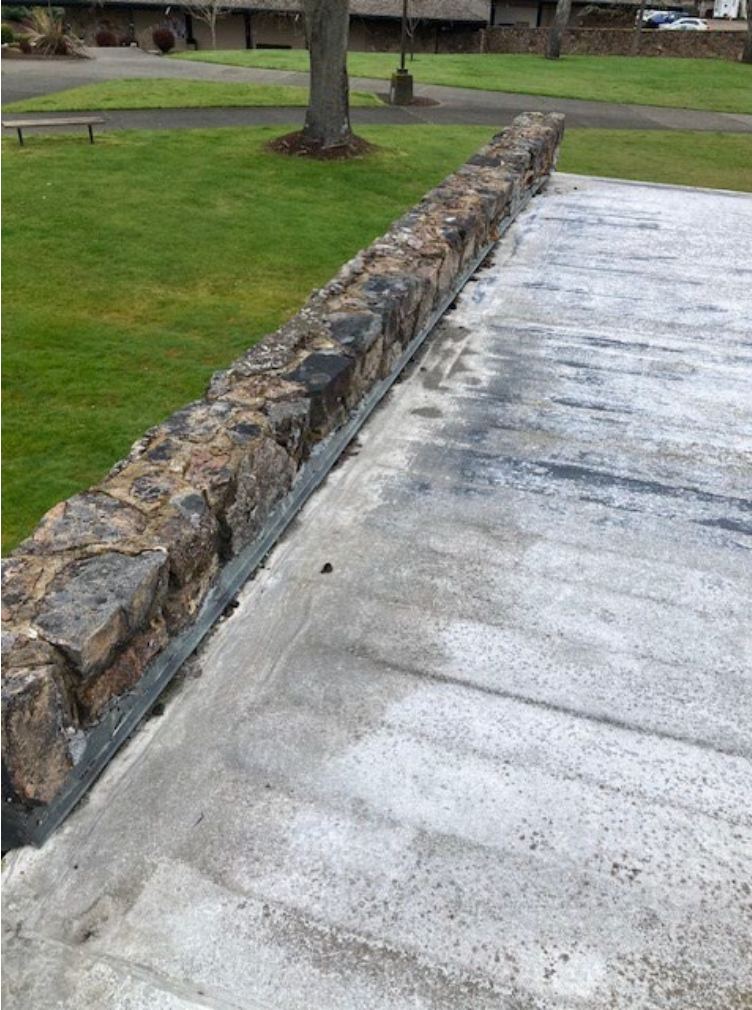
7. South Side (flat roof over offices) Rock Wall
