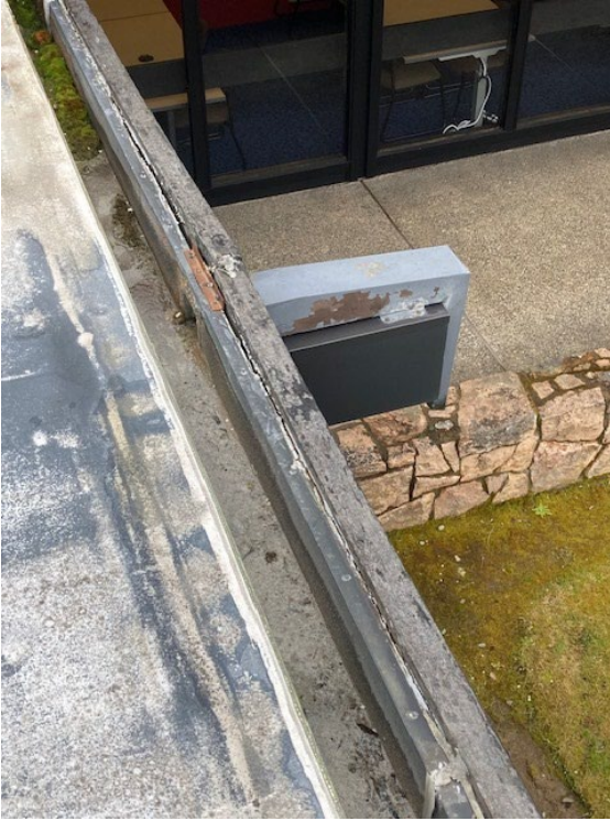
5. Gutter on South side (over offices)
